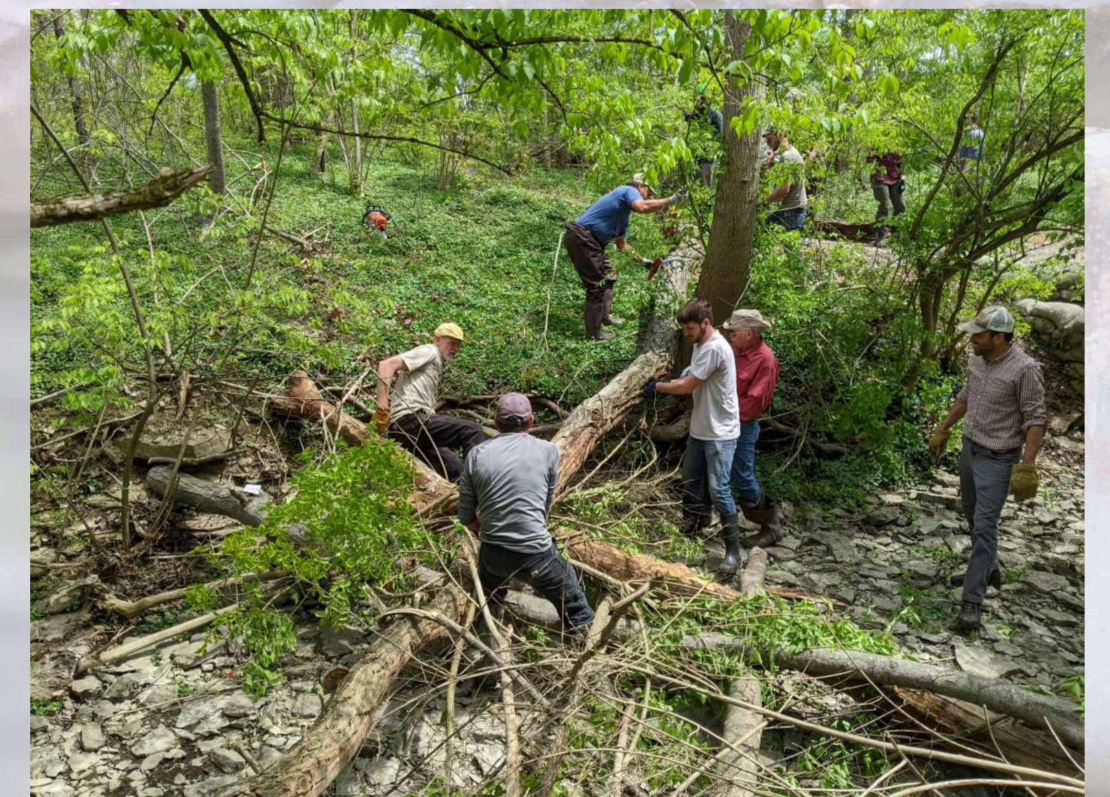
Cooper Creek Collaborative volunteers installing a hand-placed log structure just downstream of the wooden trail bridge in Bechtold Park.
